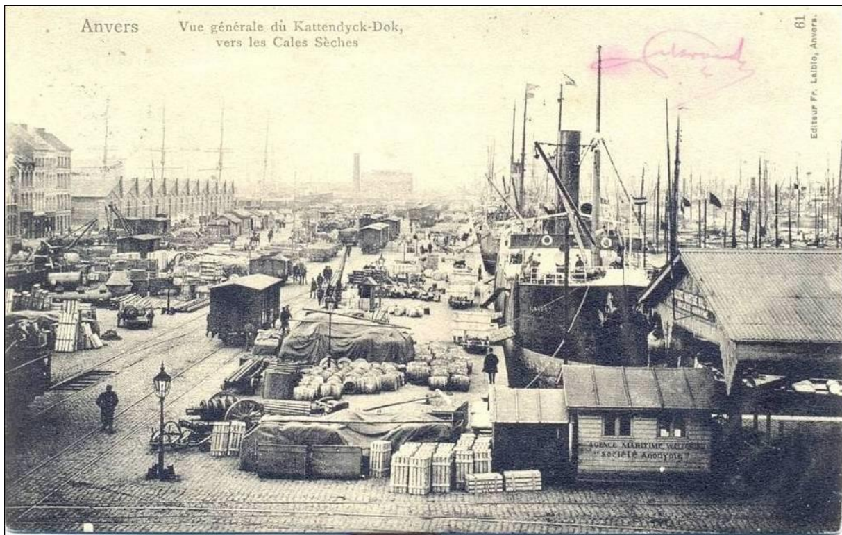
Figure 1: View of Antwerp's port, Kattendijk dock.
